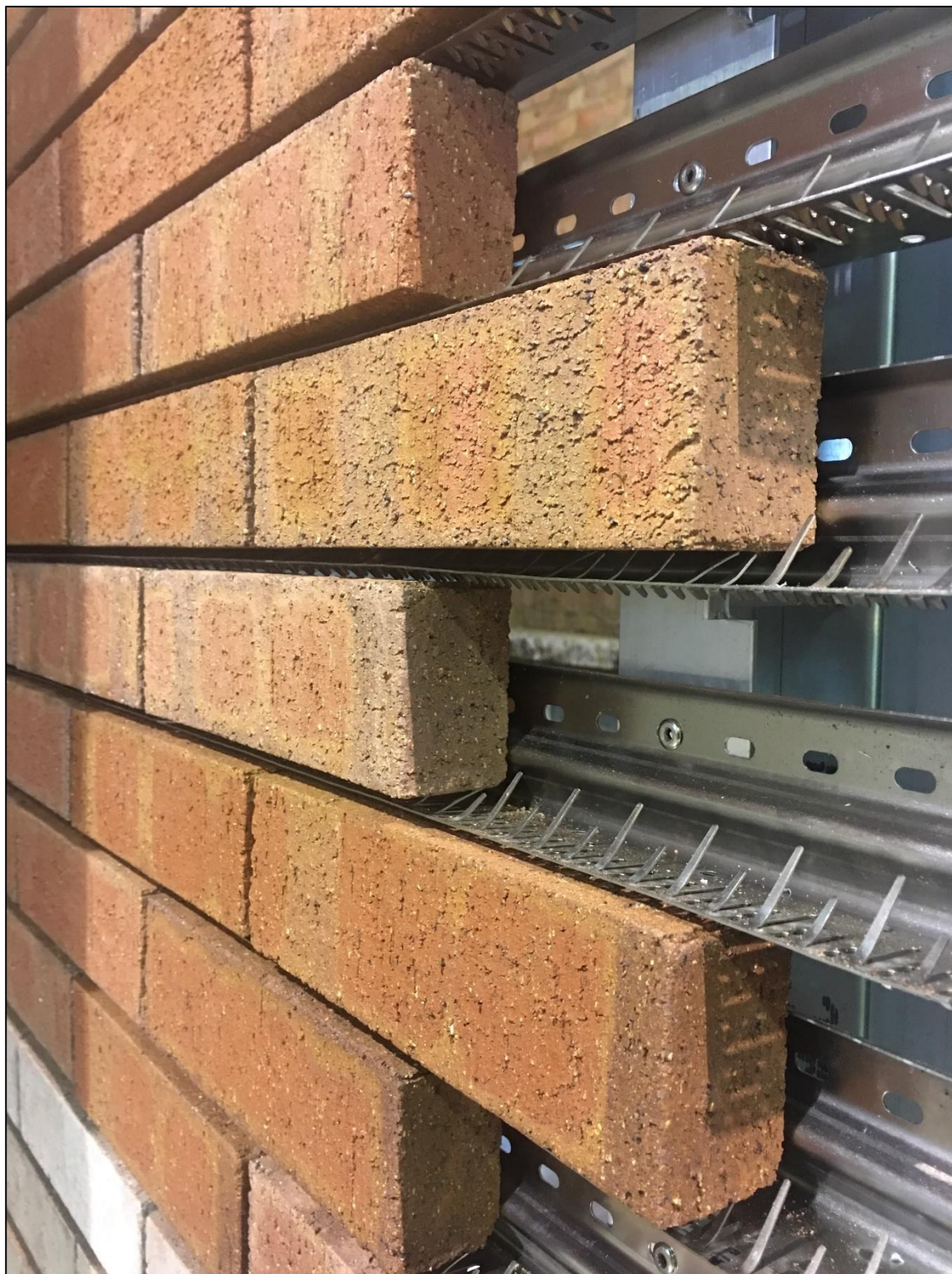
CLOSE UP OF BRICK SLIPS
